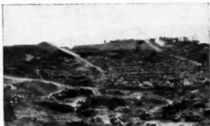
Photo by courtesy of Becker & Haag Showing Step Form of Pits in Siberian Asbestos Mines
